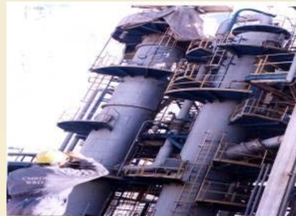
After assembling top section
