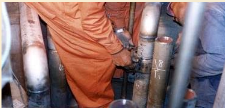
Replacing inlets and outlets of tube bundle
