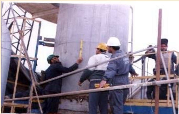
Checking fitting of new section
