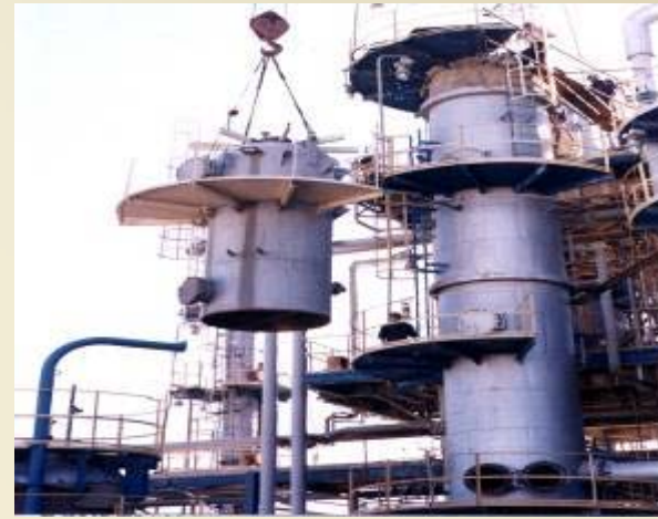
Replacing top section
