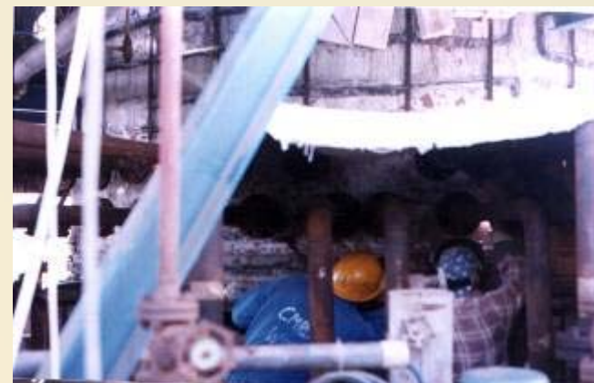
Repair welding outside of shell
