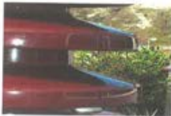
porcelain insulator for medium high voltage
